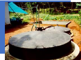
Anaerobic digester
